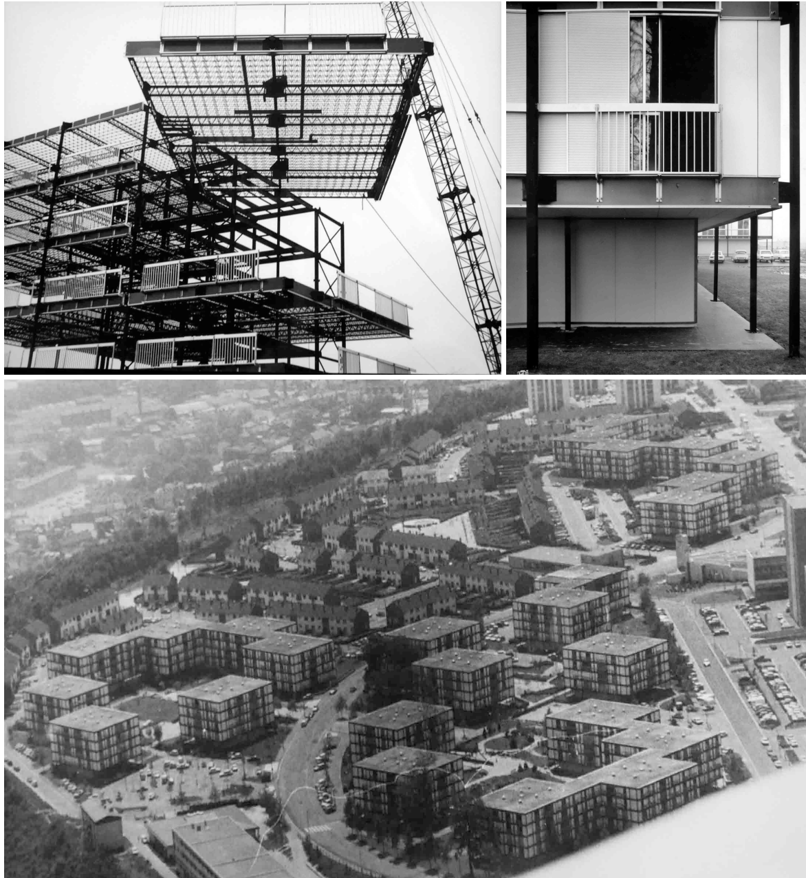
Figure 6.10: The GEAI project at Rouen-la Grand Mare by the architects Marcel Lods, P. Depondt and M. Beauclair. Top left: under construction; top right: facade detail; bottom: aerial view upon completion in the mid-1970s (Source: CAA Fonds Lods 323 AA 516/5).
