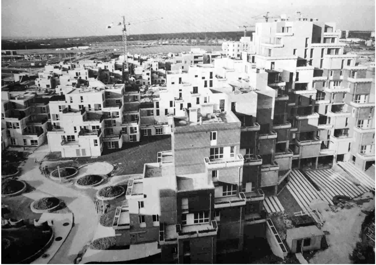
Figure 6.20: Evry I “Les Pyramides” by Michel Andrault and Pierre Parat (1971-1974) (Source: Claude Parent, “Interview, Andrault & Parat” L’Architecture , no. 403 (1977): 92-104).
