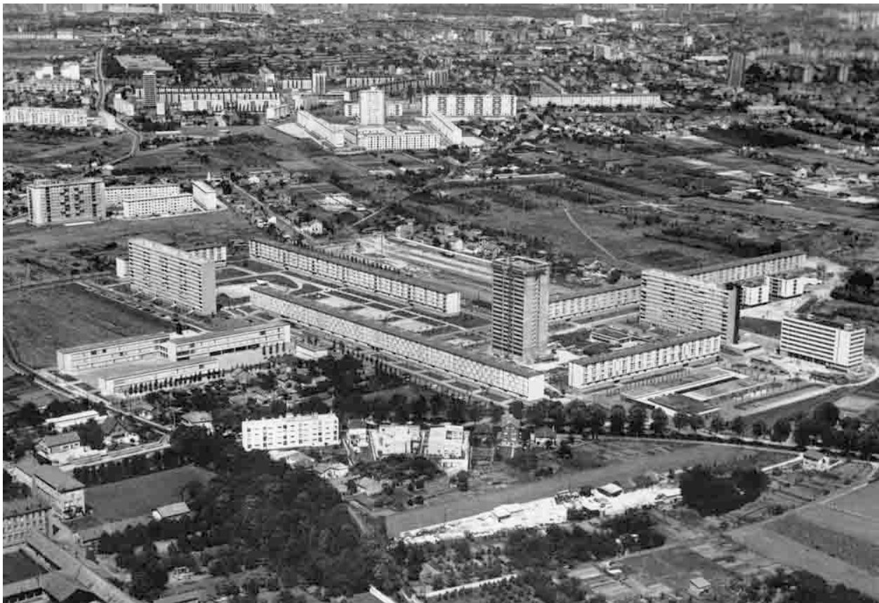
Figure 5.3: Aerial photo of grands ensembles projects in the context of the southern suburbs of Paris, as they were studied by the geographer Jean Bastié in 1964 (Source: Jean Bastié, La croissance de la banlieue parisienne (Paris: PUF, 1964): 384).
