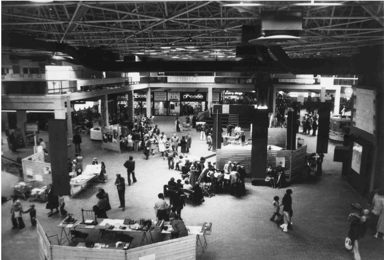
Figure 5.22: Interior plaza of the Agora of Evry. Photo taken around 1975 (Source: CAA Fonds Le Coureur, 187 IFA 44/10). Space-frame roofs like these were common features of the public architecture of French new towns during the 1970s.
