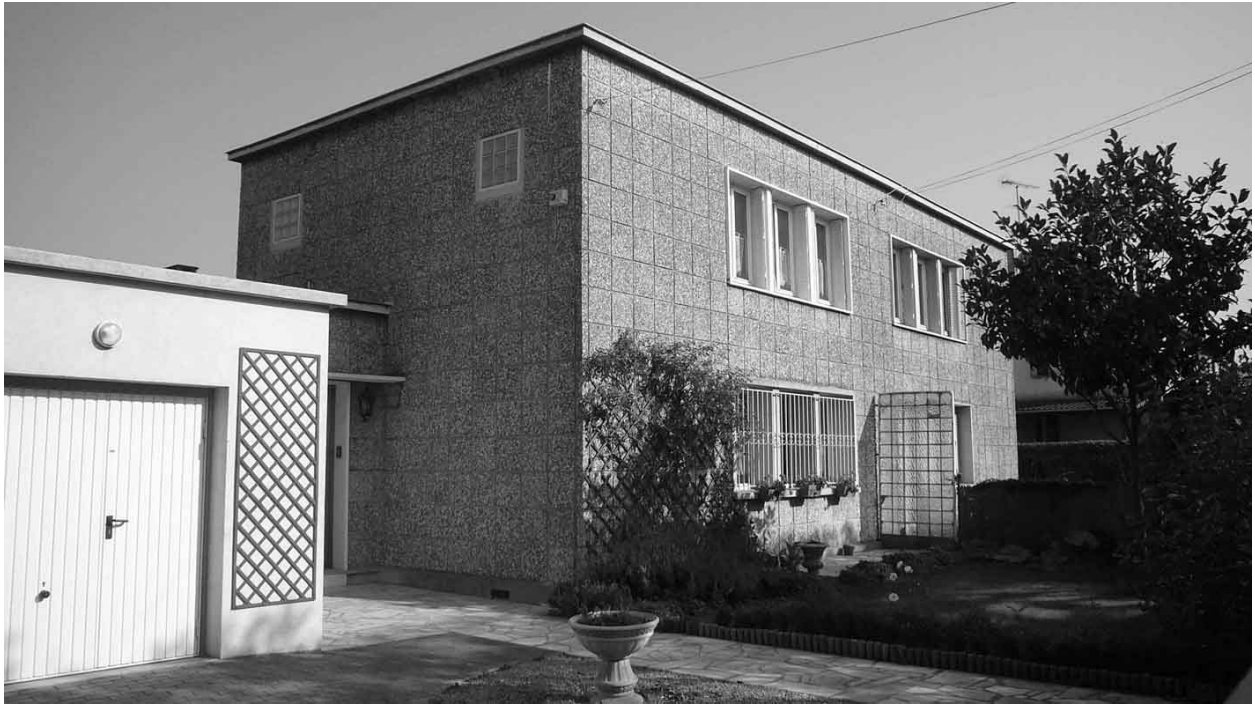
Figure 1.3: Prefabricated single-family home at Noisy-le-Sec, result of the MRU's 1946 experimental competition (photo by the author, 2008)
