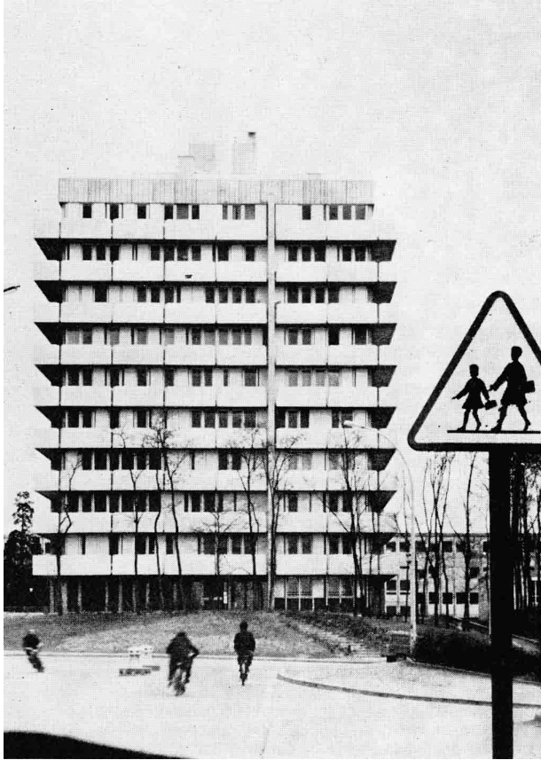
Figure 6.7: Photo around 1970 of the apartment building at Montereau by Xavier and Luc Arsène-Henry (Source: Techniques et Architecture , no. 292 “Architecture évolutive: Habitation” (1973): 94). The precast concrete balustrade elements literally overshadowed the random play of facade elements behind them.
