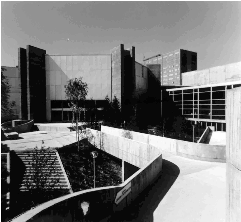
Figure 5.24: Exterior view of the Agora, photo of around 1975 (Source: CAA Fonds Le Couteur, 187 IFA 44/10). The experience of a certain blurring between inside and outside is achieved here by decomposing the program architecturally into distinct sculptural objects.
