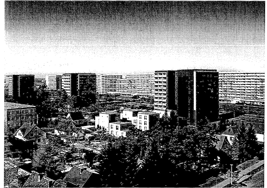
Cottbus, Plattenbau converted to detached dwellings
