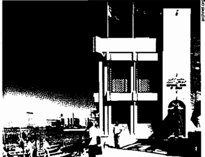
1979. National Bank of Dubai John R. Harris & Partners
