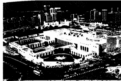
1985. Abu Dhabi Library and Cultural Center, The Architects Collaborative
