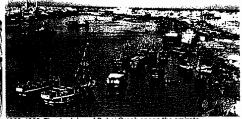
1960-1965. The dredging of Dubai Creek opens the emirate to more and larger ships and transforms Dubai into the largest port in the Gulf
